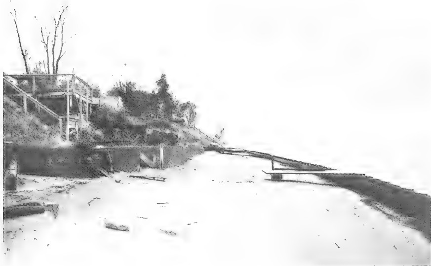
Figure 11. View southward from station 28 along the seawall (16 October 1976).
